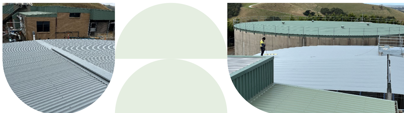
Refurbishment of Toora 1-ML CWS Tank, including new roof
