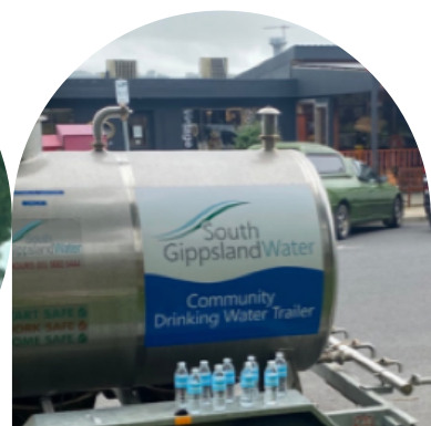
Temporary water supply trailer at Loch
